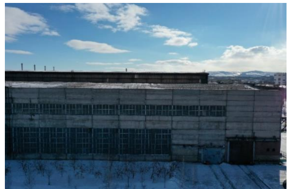
Figure 4 - Front of SLS -8 building (H-axis)
